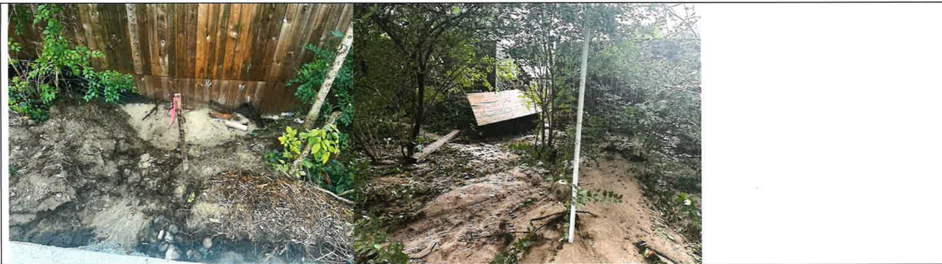
Sand base is visibly missing from under path. Later on in the day, 66 feet of concrete is removed.
